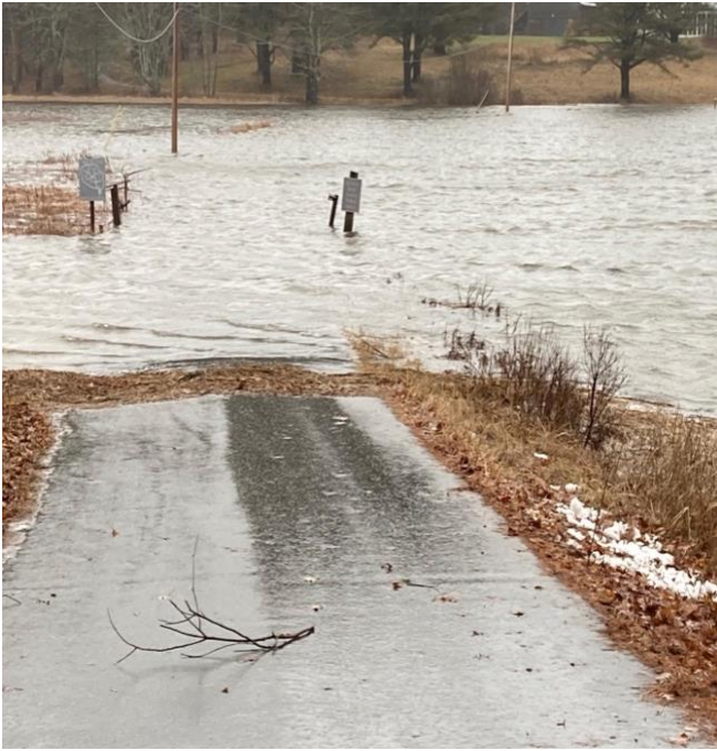
Mill Island Causeway
