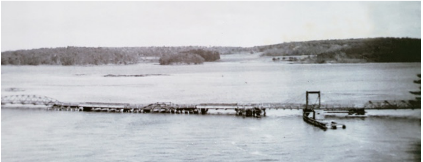
Original Arrowsic Bridge (all photos Mildred Knight)
