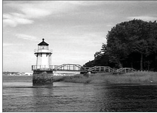
Is it 1900 or 2000? The Doubling Point Light being restored to its former historical detail.
