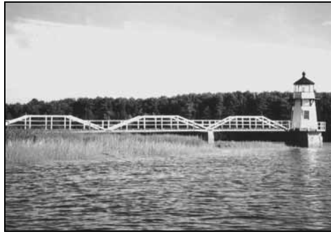
The rebuilt and painted walkway at the Doubling Point Light.
