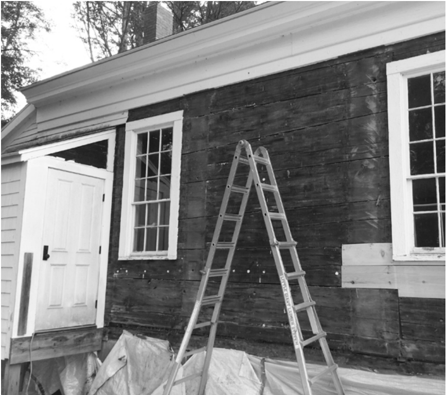
Prepping Town Hall north wall for siding
