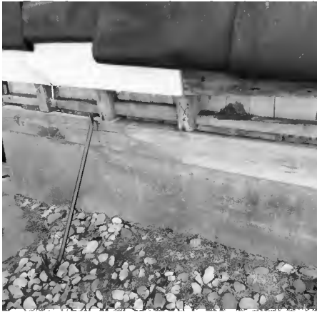
Skillful sill repair (left) and damage to be repaired (right)
