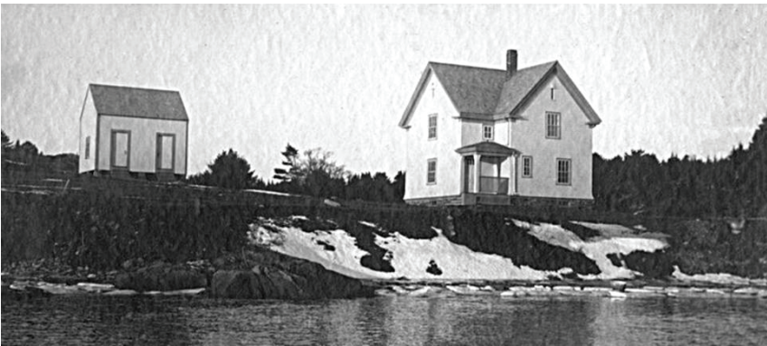
Range Lights Keeper's Quarters and Privy Barn, circa 1899
