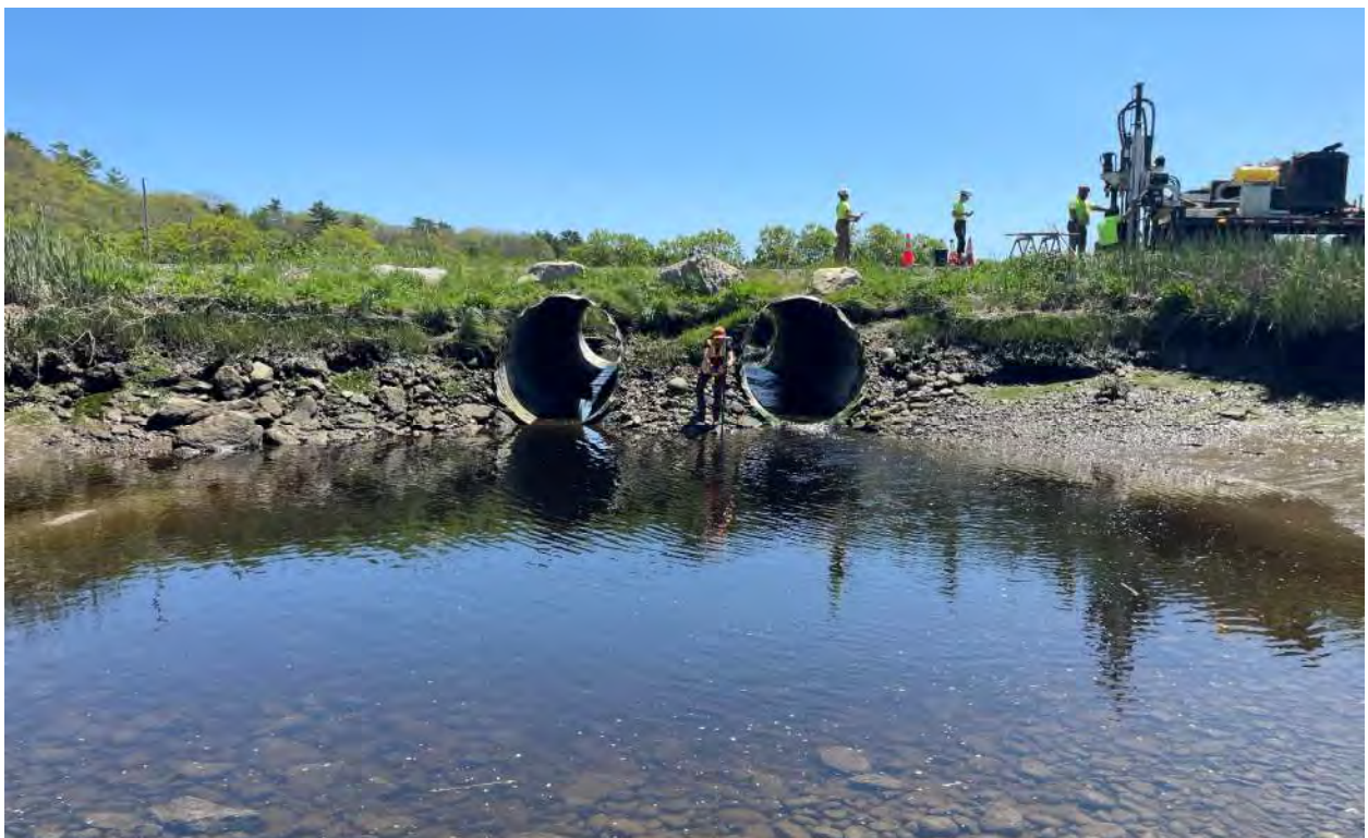
Figure 5. Photo of Spinney Mill Road Crossing twin corrugated metal culverts. View of downstream end of culverts at low tide.
