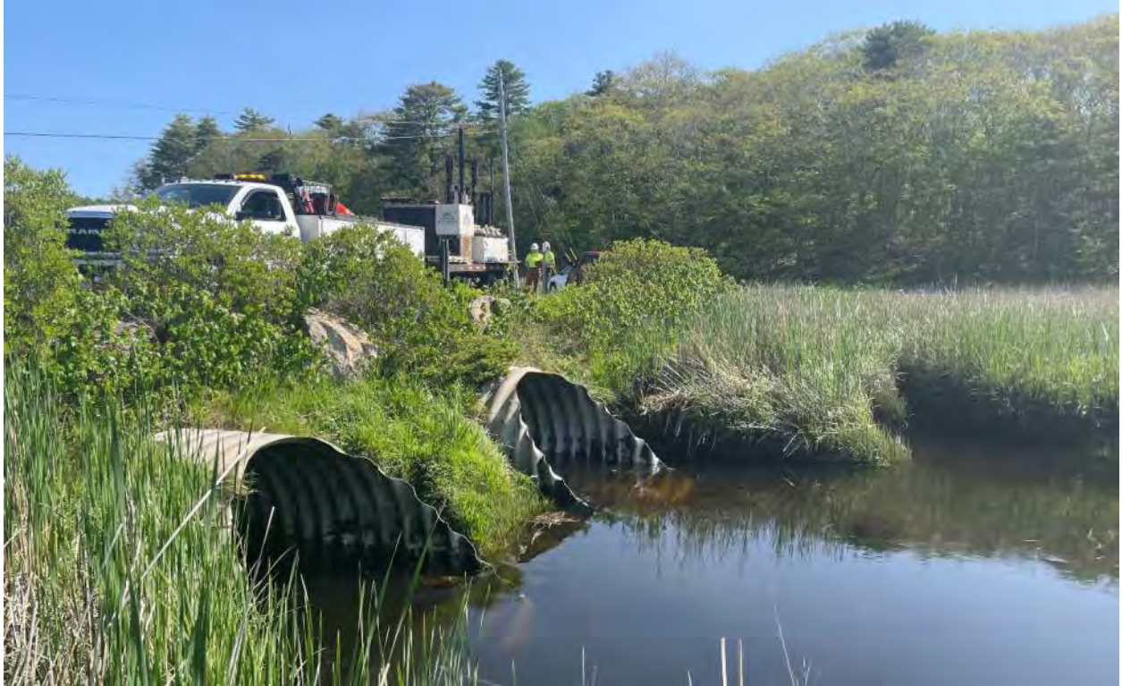
Figure 4. Photo of Spinney Mill Road Crossing twin corrugated metal culverts. View of upstream end of culverts at mid tide.
