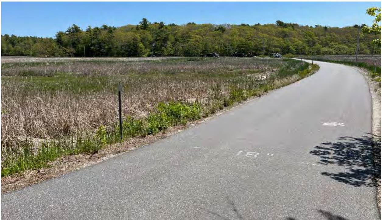
Figure 7. Photo of Spinney Mill road crossing the marsh, looking east. Note numbers painted on the road to indicated depth over the center of the roadway during road overtopping events.
