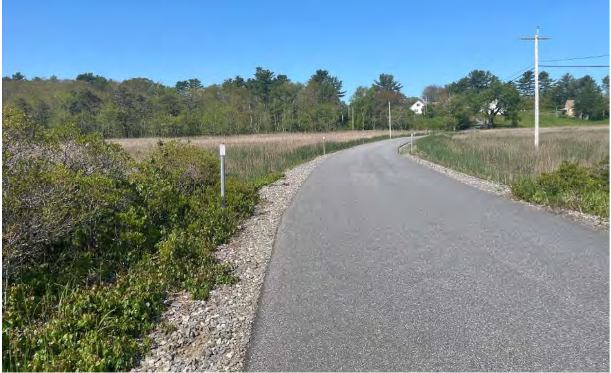
Figure 6. Photo of Spinney Mill road crossing the marsh, looking west.
