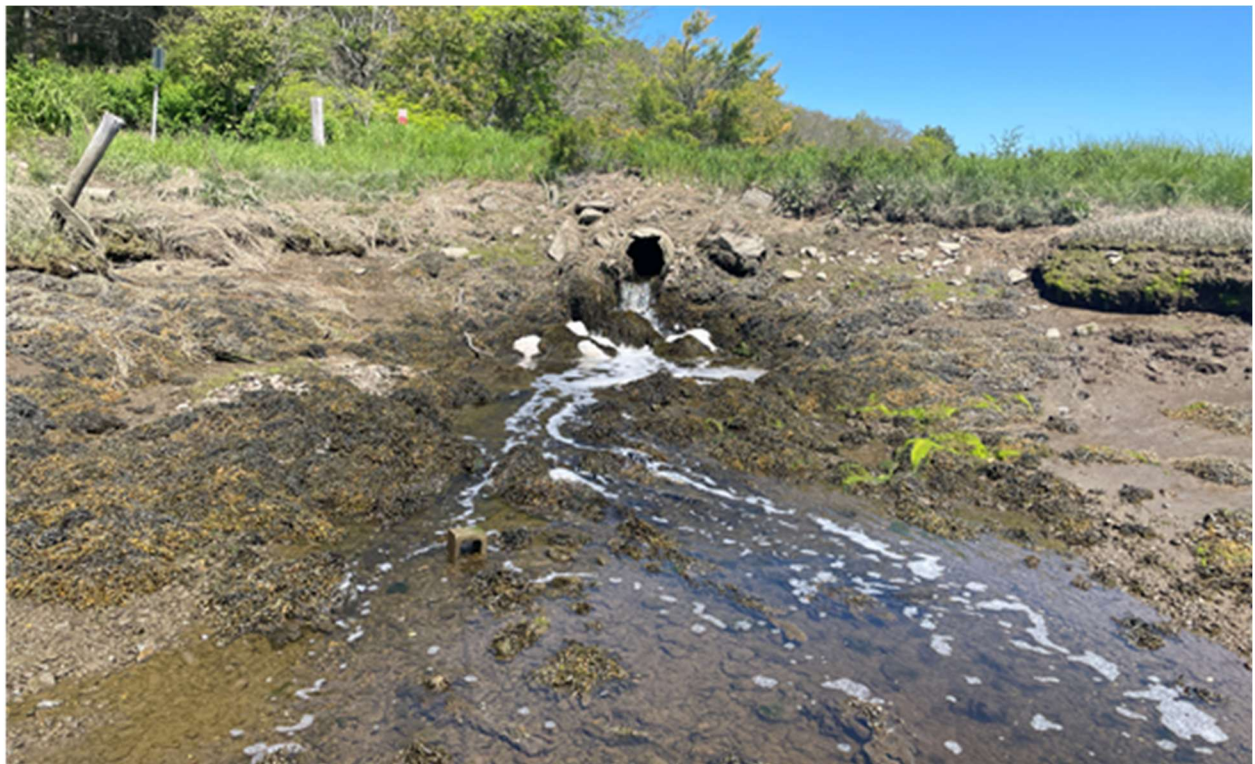
Figure 5: Existing culvert under Indian Rest Rd, looking north.
